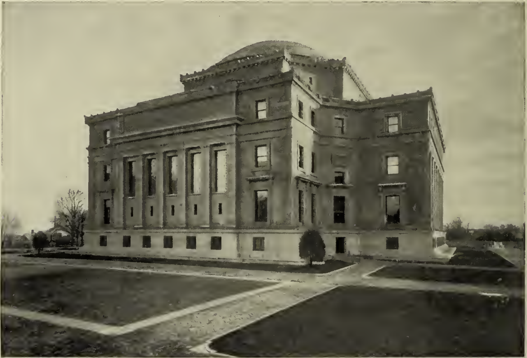
LAW SCHOOL WING OF LIBRARY BUILDING
